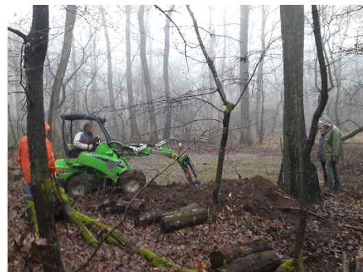
Fig 2b. Trench digging with BobCat trencher
