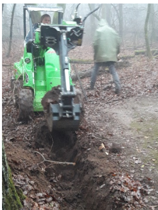
Fig 2a. Trench digging with BobCat trencher
